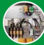
The voltage regulator is protected by a circuit breaker with magneto thermal release. The auxiliary circuit is protected by fuses.
